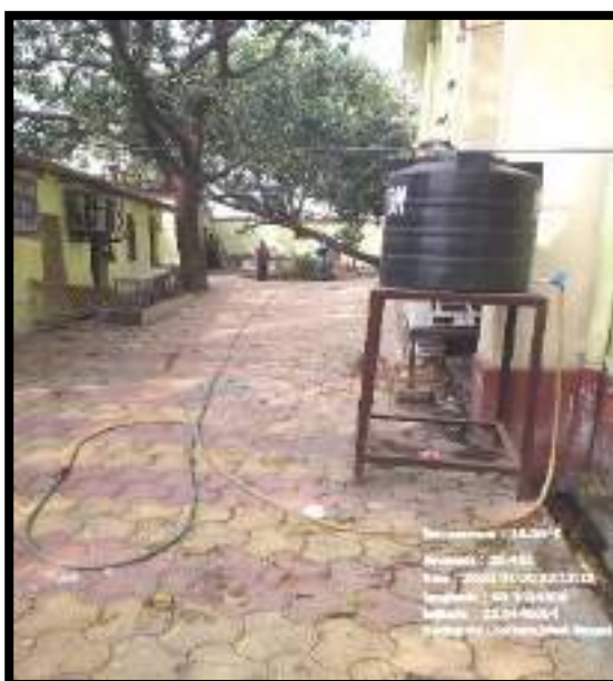
Recycling of Condensate from Air Conditioner
